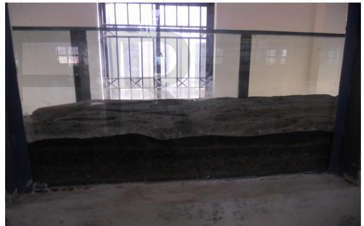
Fig. 4.b U/S Sediment profile after Flushing Grid no.3, 4, 5, and 6
